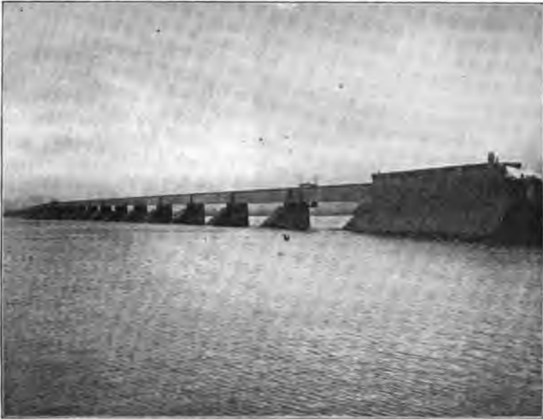
Old Victoria Tubular Bridge Over the St. Lawrence, Grand Trunk Railway, Montreal, Canada
