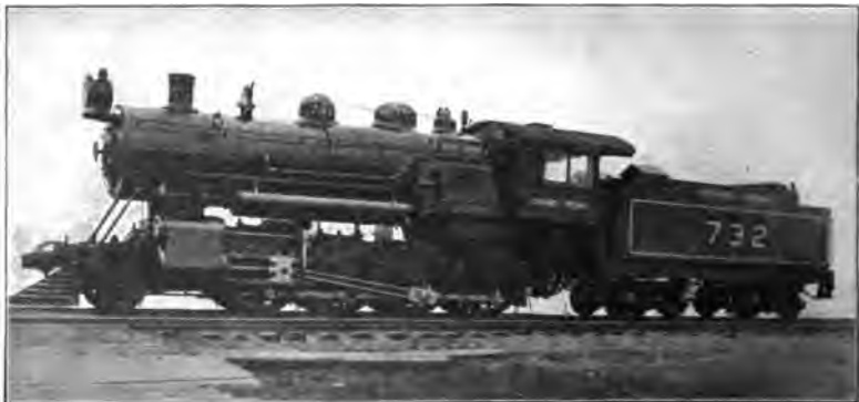
Modern 2-8-0 Compound Freight Engine, Built by Grand Trunk Railway, Montreal Shops. Cylinders, 22½ and 35 x 32 Inches; Drivers, 63 Inches Weight of Engine, 211,200 Pounds
