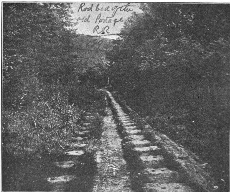
Ruins of Old Portage Roadbed
